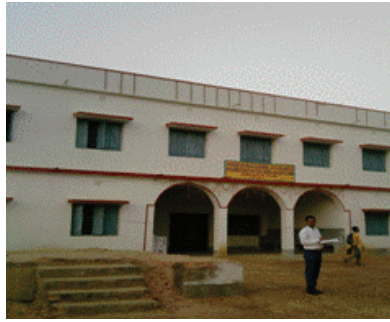
Construction of SC/ST Hostel building at Chandra
