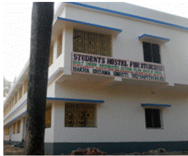
Construction of SC/ST Hostel building at Dasbandh
