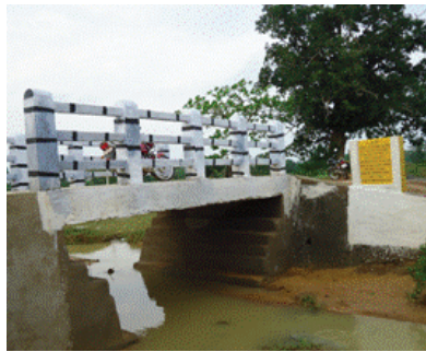
Construction of culvert at Lalgarb
